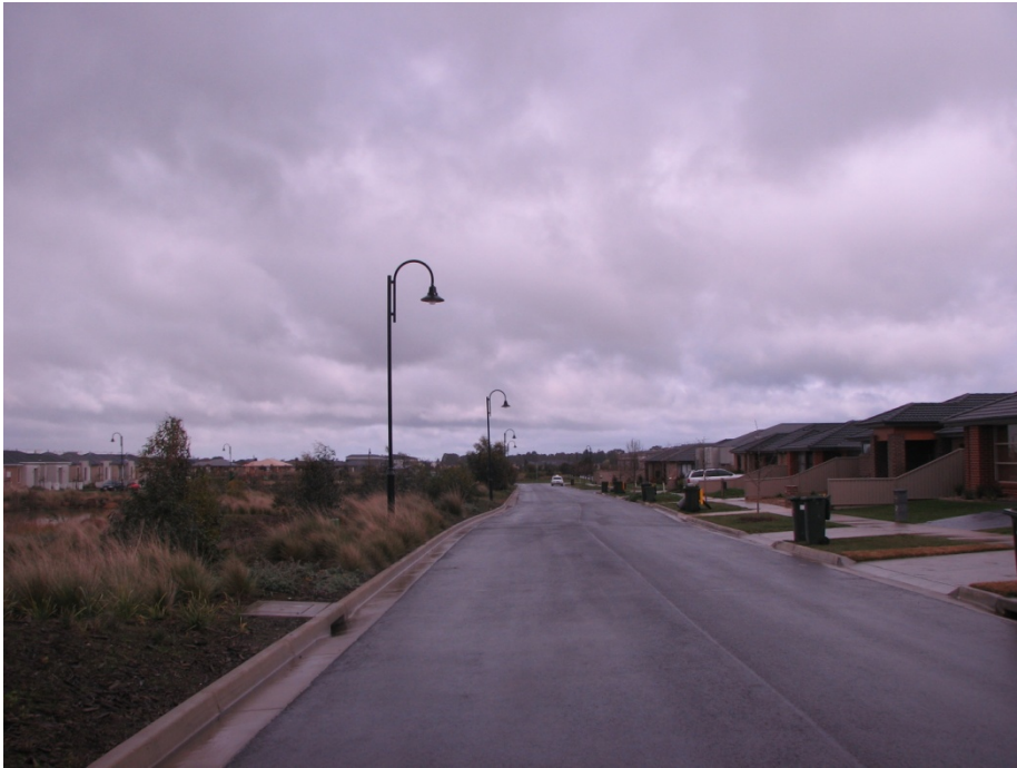
Fig 7. This type of light is lower and has a shade to reduce spill lighting, it is located on Jarrah Drive in Alfredton, Victoria. They are only on one side of the street and overall there is reduced light spill and environmental impact.
