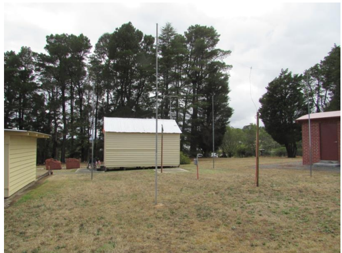
(Above) The Radio aerial array and restored Radio Shack.
